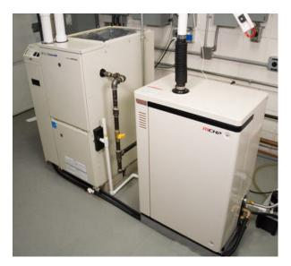
Combined with heat storage a flexible device for electricity production
